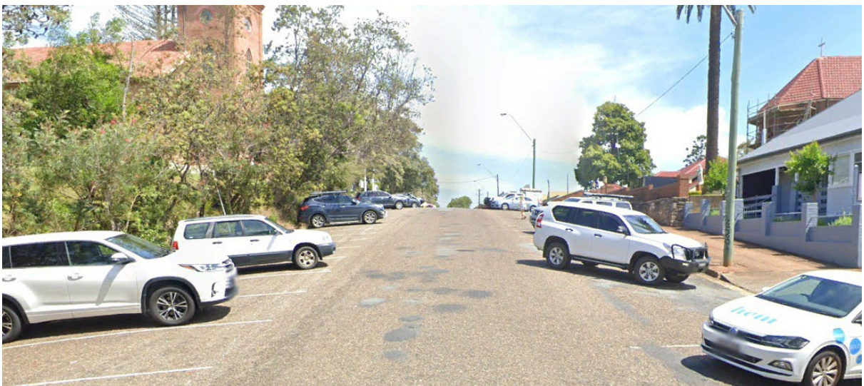
Figure 31 Looking south on Hay Street (Google Earth Pro)
