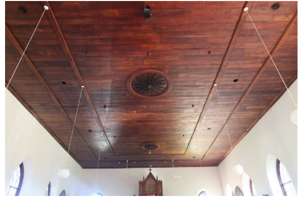
Figure 61 View of church ceiling. Source: Author
