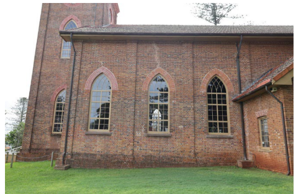
Figure 53 View of windows on south elevation. Source: Author
