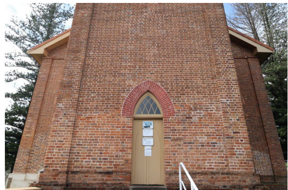
Figure 40 View of door on west elevation. Source: Author
