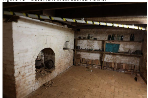
Figure 75 Basement area. Source: Author
