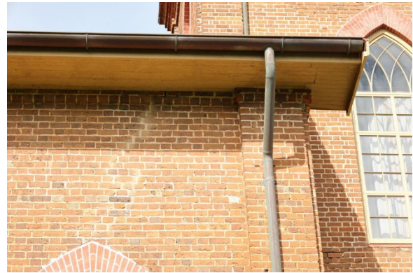
Figure 47 Detail of brickwork condition on north elevation. Source: Author
