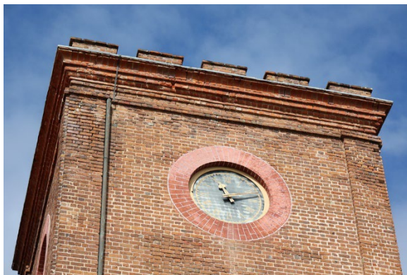
Figure 39 View of tower. Source: Author
