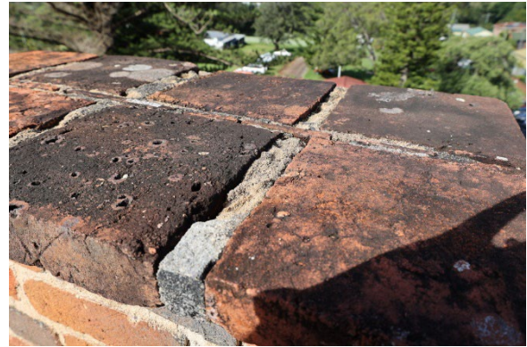
Figure 42 Detail of brickwork condition in tower. Source: Author
