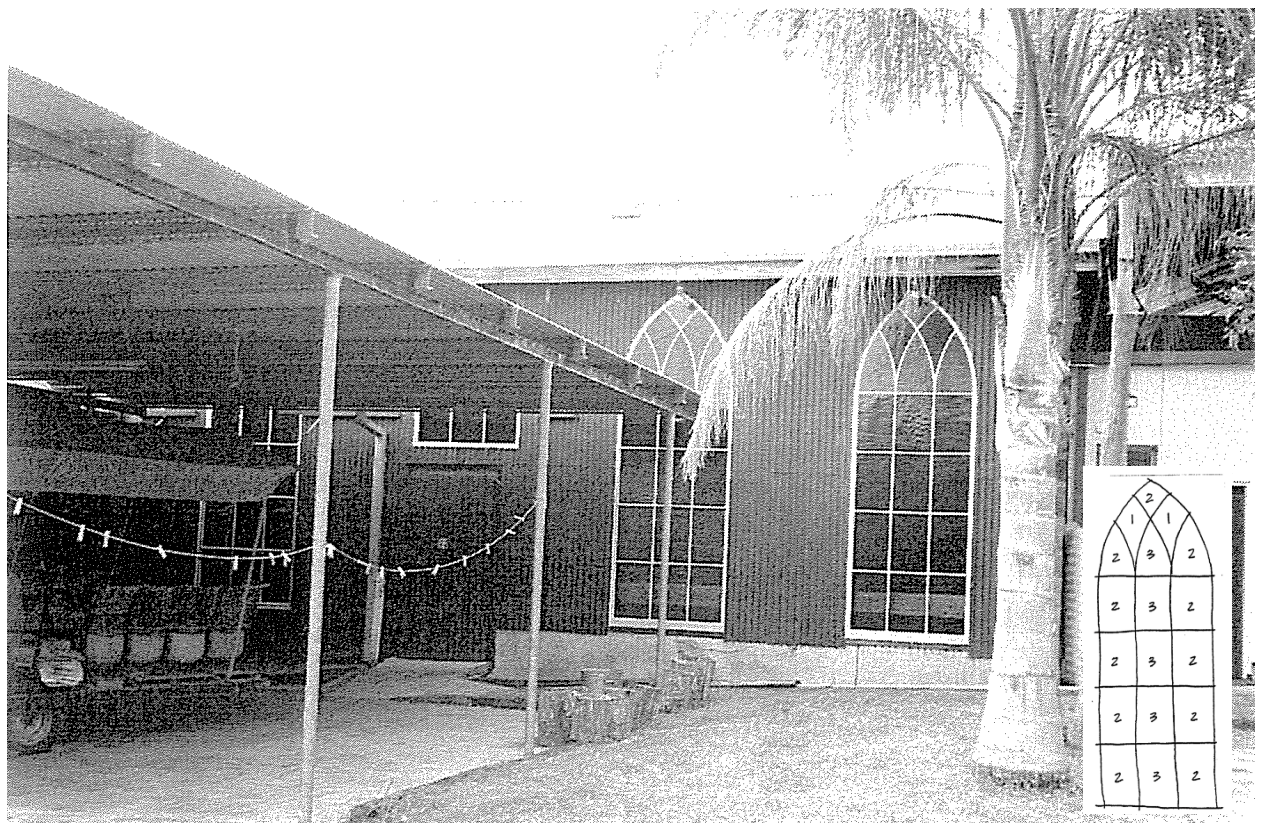
Figure 17 Former St Thomas' lancet windows in place at The Old Butter Factory Telegraph Point, NSW. Sketch of windows existing in The Old Butter Factory, indicating colour: 1 – ruby red, 2 – blue, 3 – amber. Source: Suters Architects.
