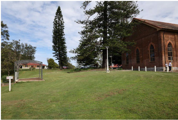
Figure 49 View of eastern elevation and adjacent grounds. Source: Author
