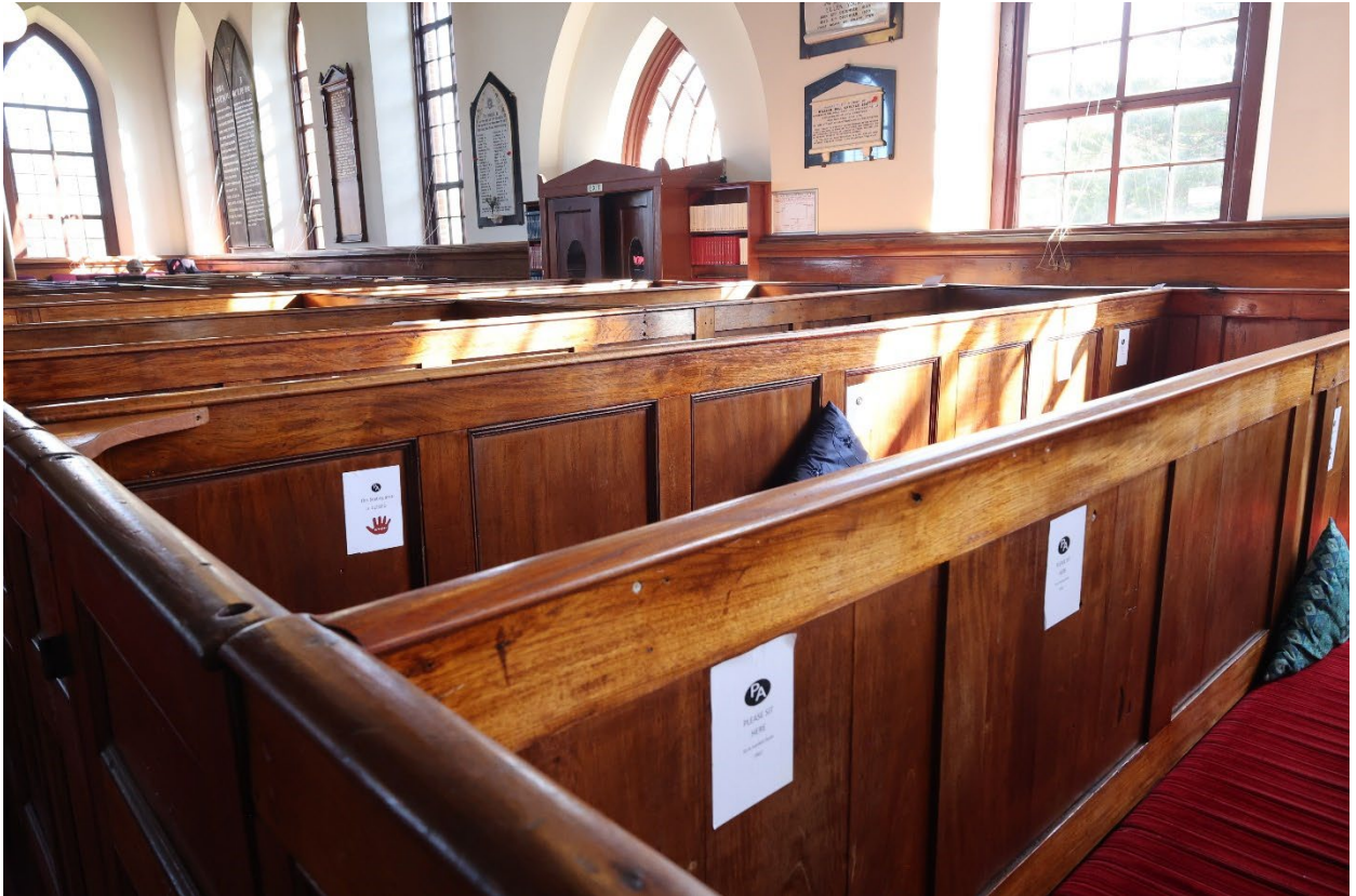
Figure 65 Restored pews. Source: Author.
