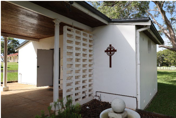
Figure 34 View of passageway area. Source: Author
