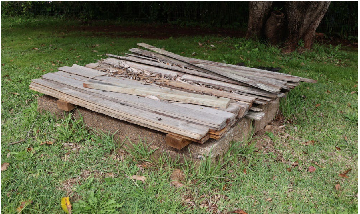
Figure 69 Location of former well at the rear of residence. Source: Author
