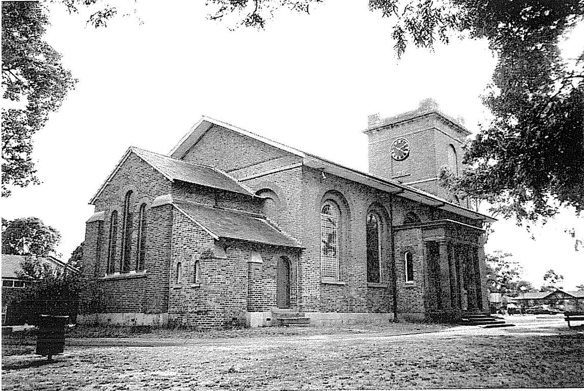
Figure 84 St Luke's, November 1998. Source: Suters Architects.
