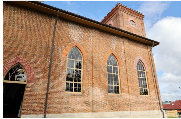
Figure 45 View of windows on north elevation. Source: Author
