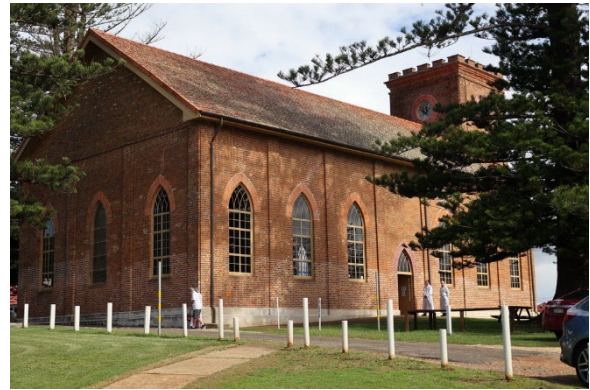
Figure 50 View of northern and eastern elevation. Source: Author
