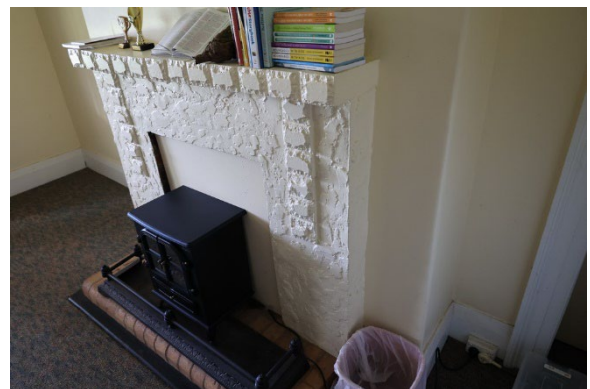
Figure 71 View of interior office areas of building showing previous works. Source: Author
