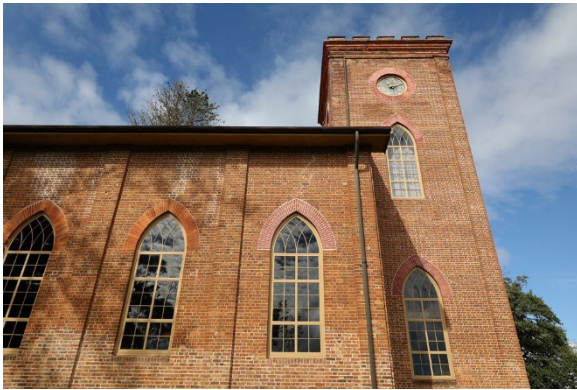
Figure 46 View of tower from northern side of the building. Source: Author
